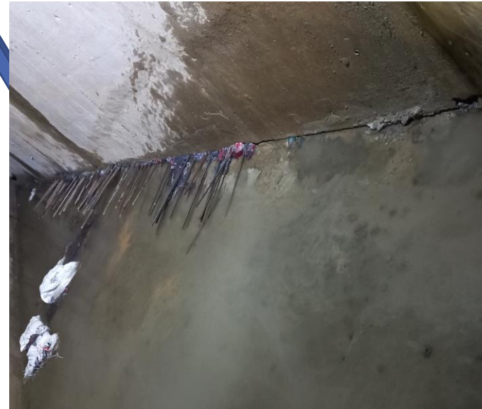
Sealing by foam inside and rugs by outside
