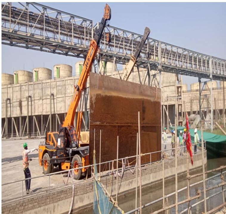
Fixing of 20 mm plate on the interconnection wall section.
