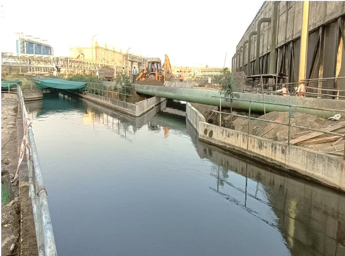
Interconnection of New Cold water channel with Existing Channel of Rihand Stage III
