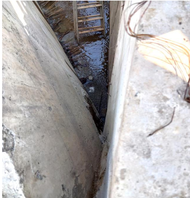
Water filled in adjacent segment of channel to avoid risk of brick wall failure.
