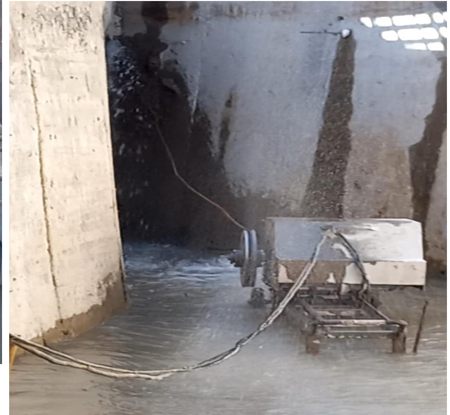
Water filled in adjacent segment of channel to avoid risk of brick wall failure.
