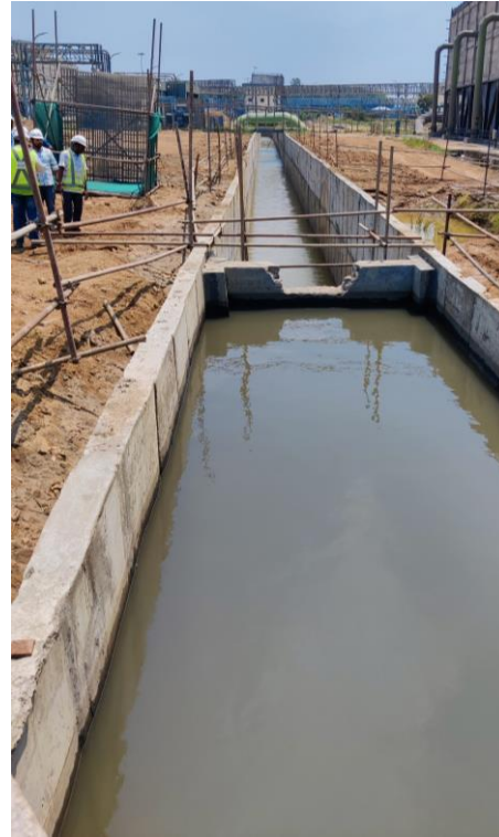
Water filled in adjacent segment of channel to avoid risk of brick wall failure.
