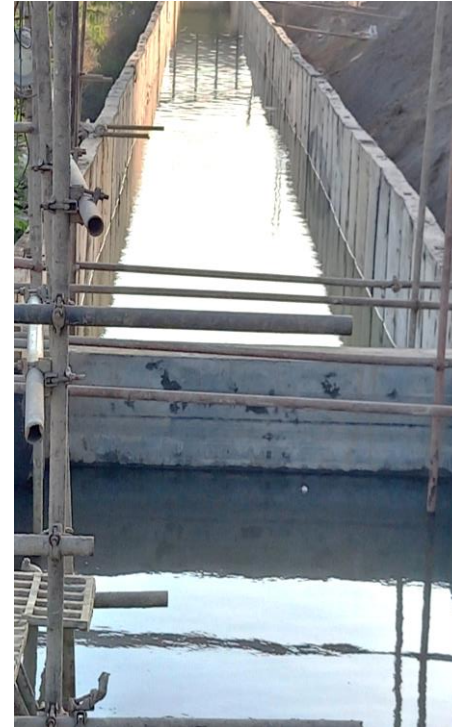
Water filled in adjacent segment of channel to avoid risk of brick wall failure.
