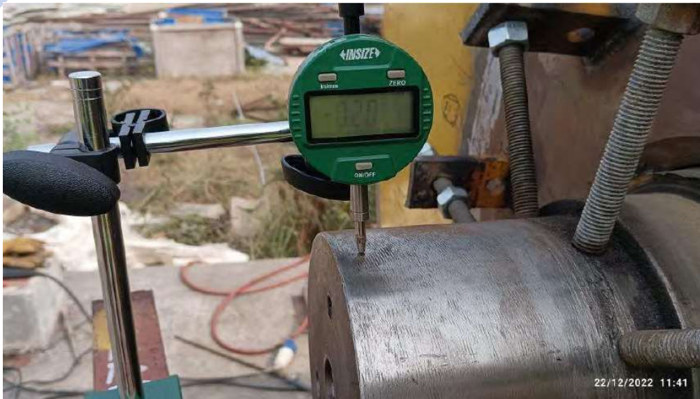
8. Dial gauge used for checking of alignment of shaft Centre with hole center.
