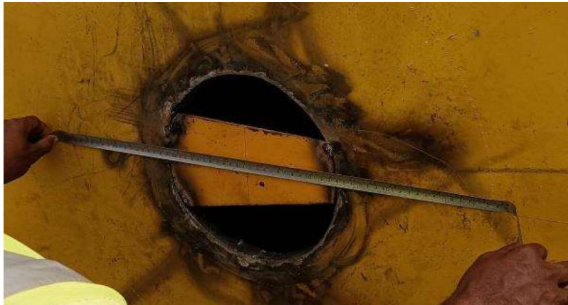
4. Centre marking on NDS outer flange.
