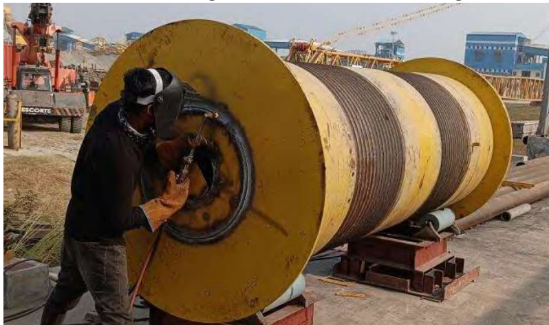
Cutting of NDS outer diaphragm for Fixing of Plate 1A
