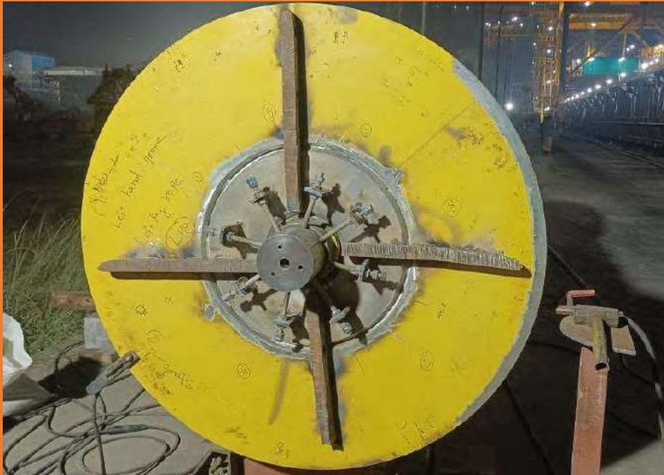
10. Stiffeners used for final fixing of outer plate
