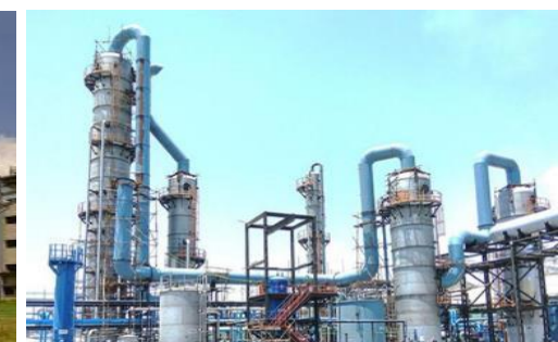
Carbon Capture plant, Vindhyachal
