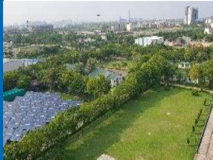
NETRA Solar PV
