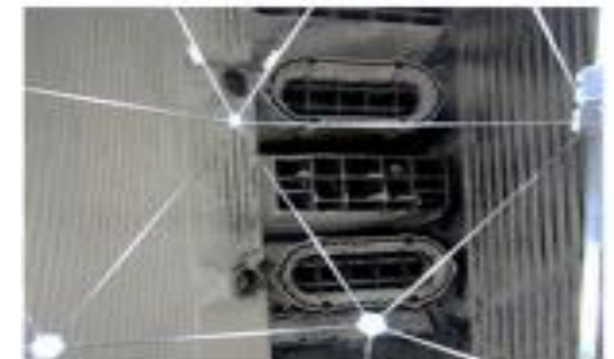
Burner section inspection
