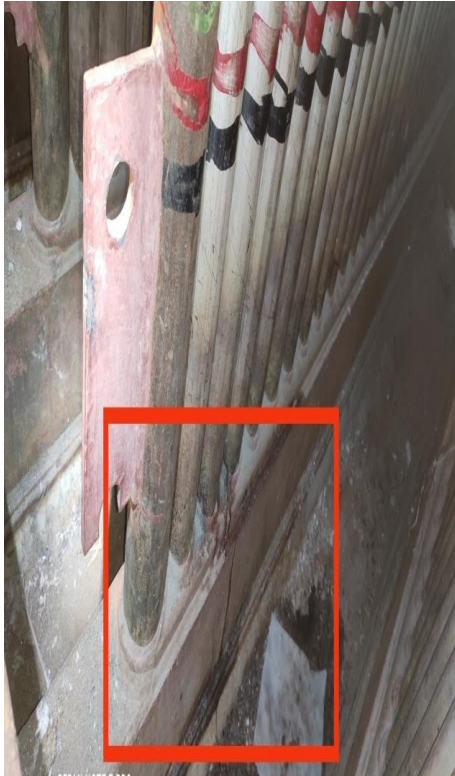
Shop Welded Joints
