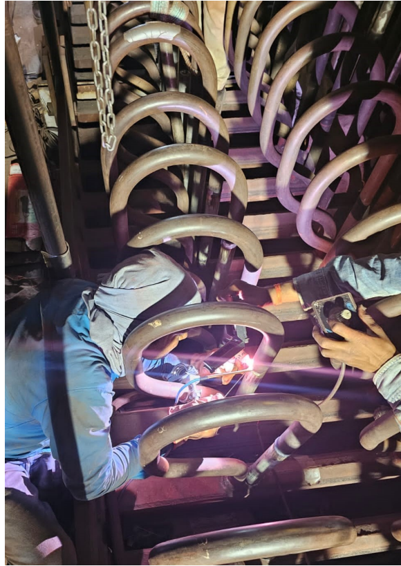
Welding of after inserting Spool
