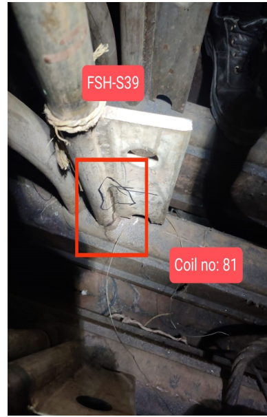
Seepages observed in Shop welded attachment lifting lug joints & Roof Seal band area in Finish Superheat (FSH) inlet Super 304H coils (S-39) of during 1 st Hydrotest
