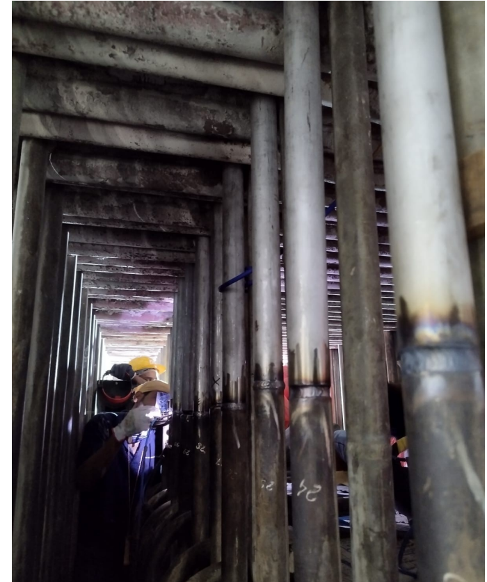
Below Roof Spool welding in progress
