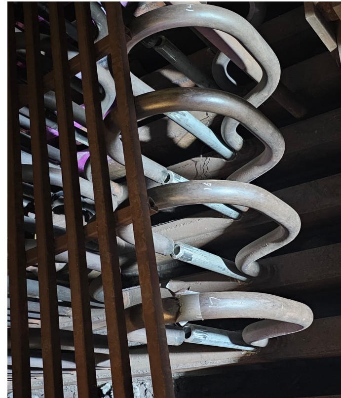
Inserted new spool tube
