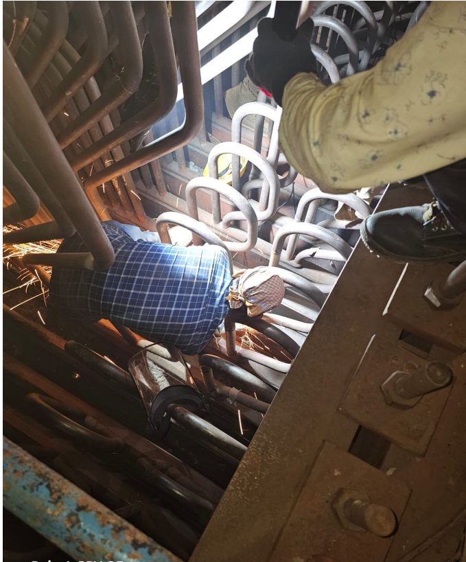
Cutting for removal of 1 st tube
