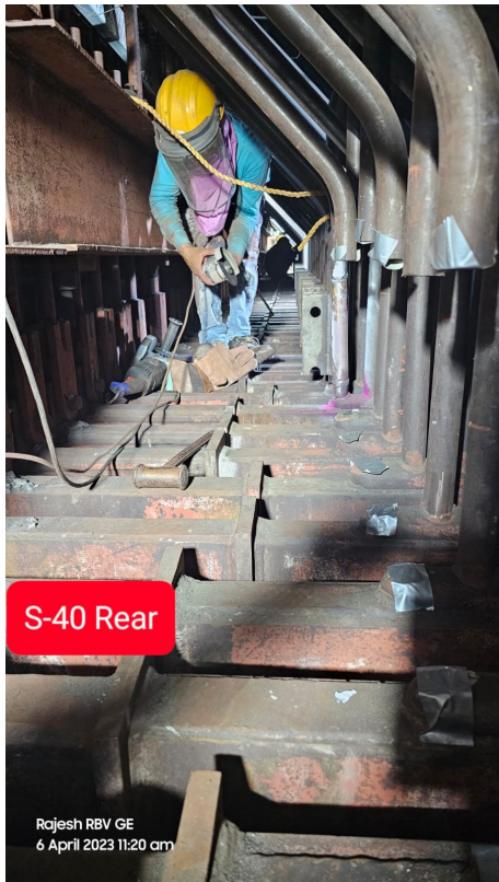
Cutting for removal of 1 st tube
