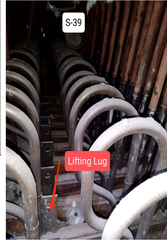
FSH INLET COILS (S-39) REAR
