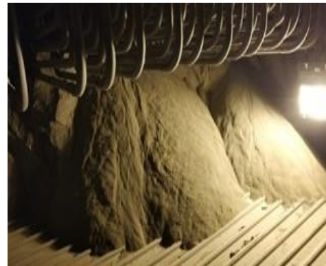
Ash Deposition at Low Loads
