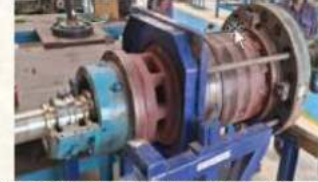
(Figure 4. Overhauling of Cartridge at Vadodara RES)
