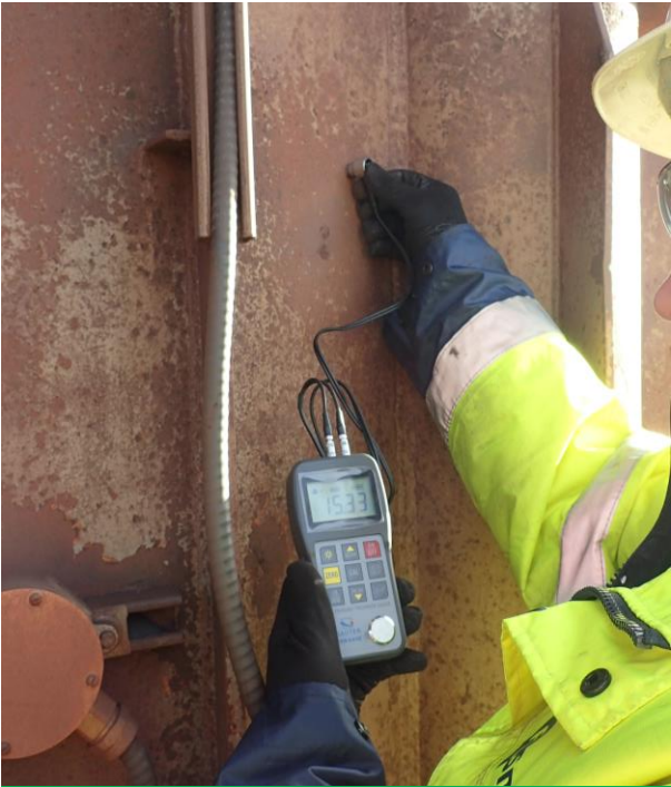
Initial Audit & Detailed Inspection
