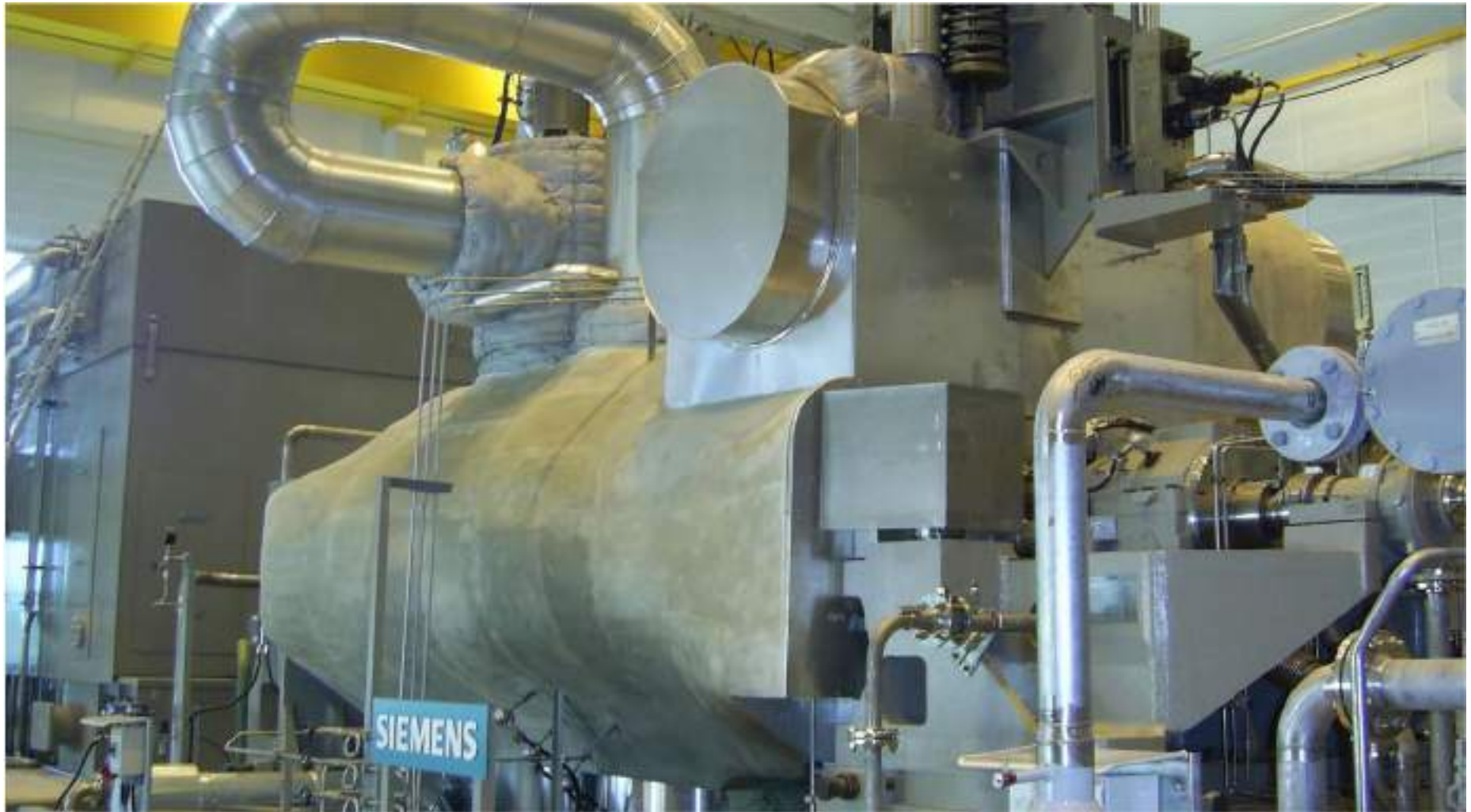
Spray insulation on steam turbine
