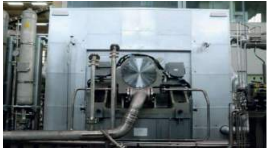
Completed enclosure with cover sheets and heat retention shield
