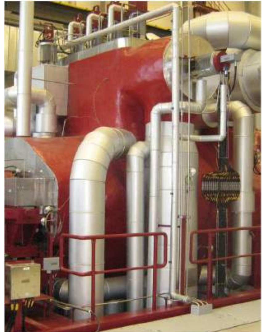
Spray insulation on steam turbine
