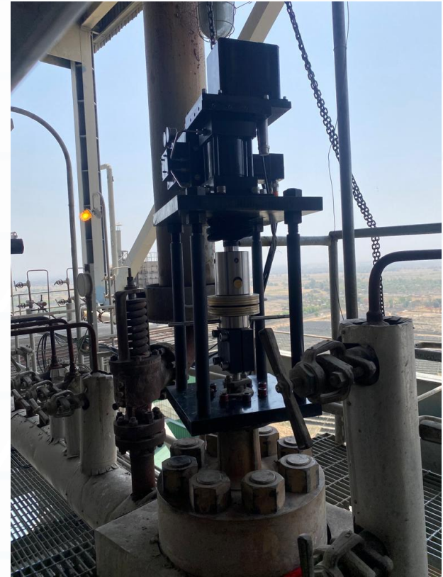
After (KSB MIL valve with REXA's Actuator)
