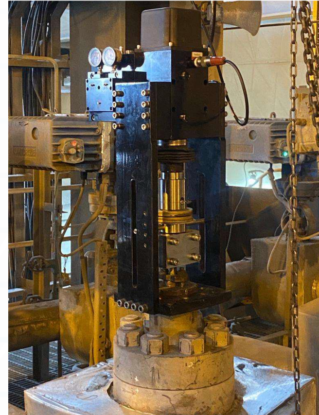
After (KSB MIL valve with REXA's Actuator)
