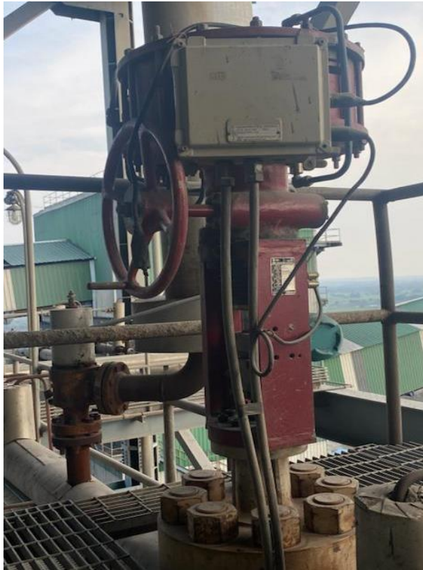
Before (KSB MIL valve with Pneumatic Actuator)
